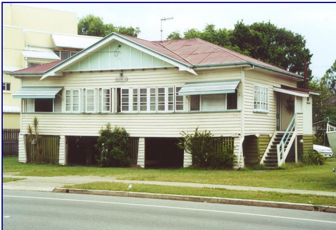
"Shieldston Flats" as it now appears.
