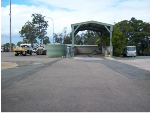
Minor servicing facility at Council depot
