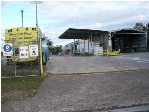
Maintenance facility at Marcoola depot
