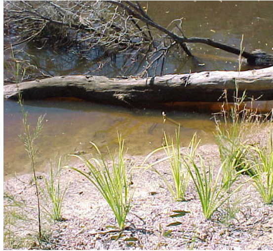
Figure 15-1 Native grasses used to stabilise creek bank
