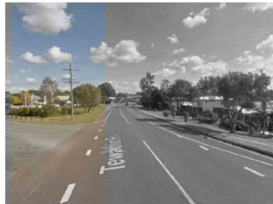
Localised View along Tewantin Road to RSL Park/ war memorial/ Diamond Street
