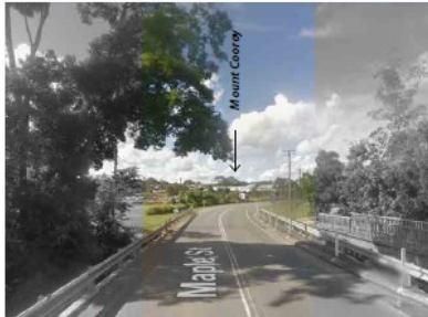
Contextual View from Cooroy Creek Bridge to Mount Cooroy (with Library and Butter Factory)
