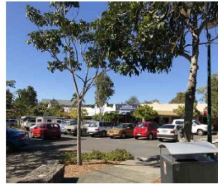
Localised View - down Memorial Avenue, low scale buildings follow the topography down the hill, marked by the 2 storey Pomona Hotel at the low
