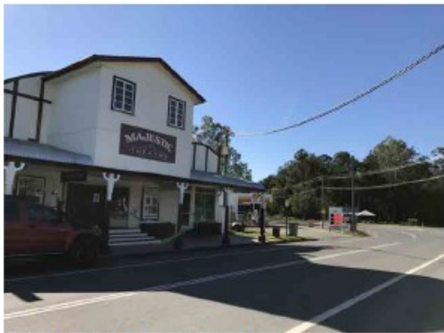
Localised View - to Majestic Theatre (Heritage Qld register)
