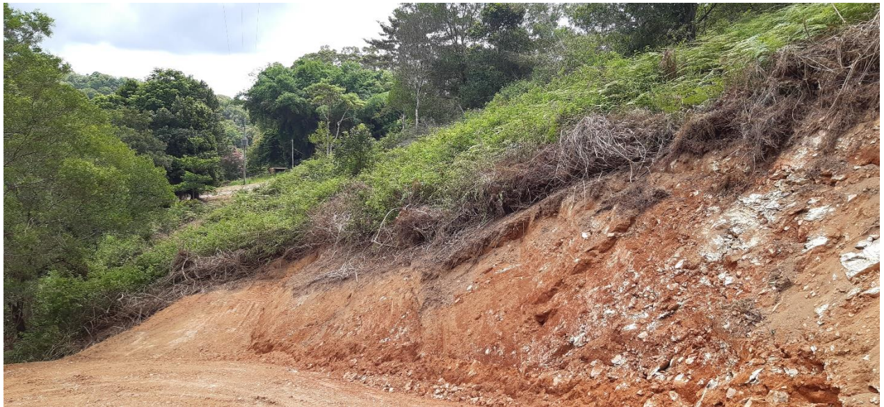
Figure 3 – Bend at the bottom of access track
