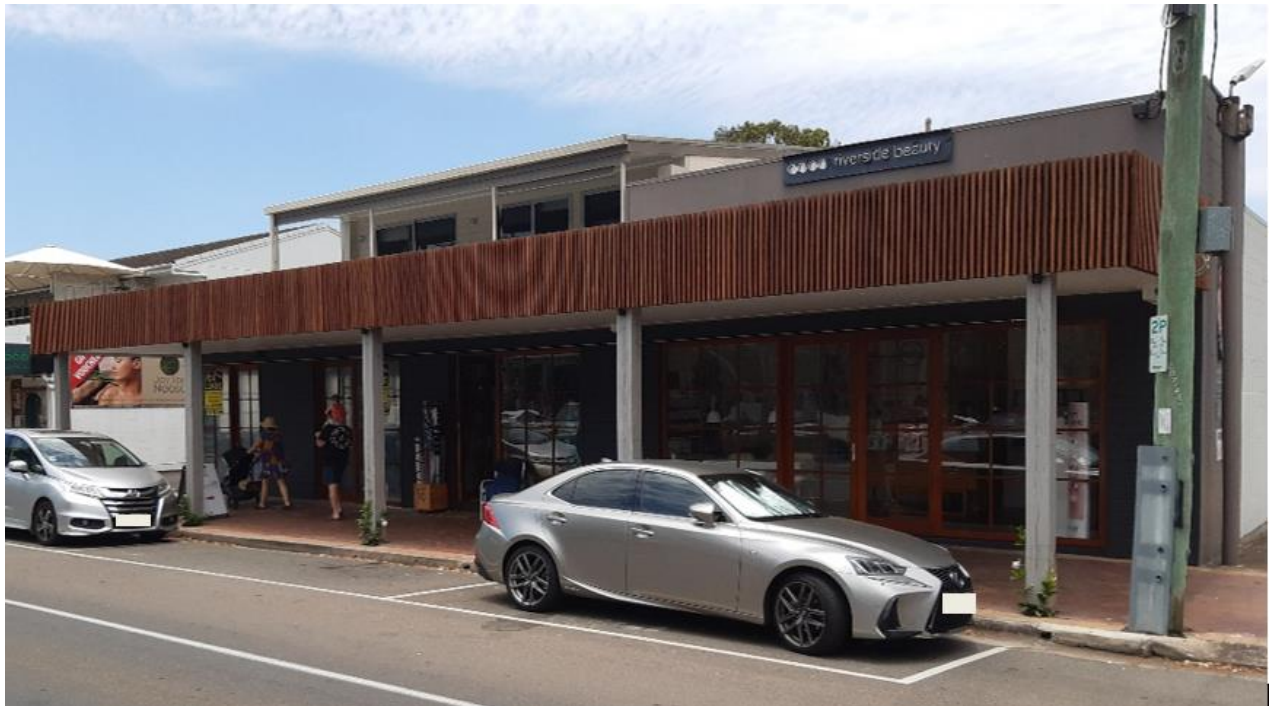
Figure 3: Updated awning along western elevation of 6 Thomas Street
