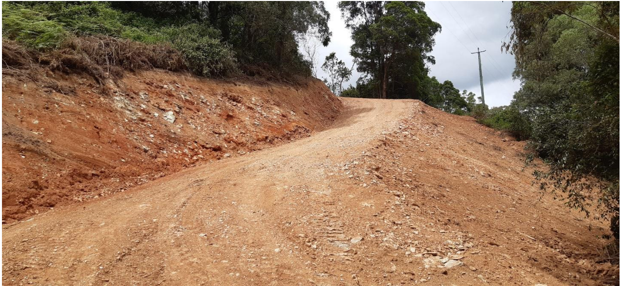
Figure 2 – Freshly cut access track in Landslide Hazard Overlay
