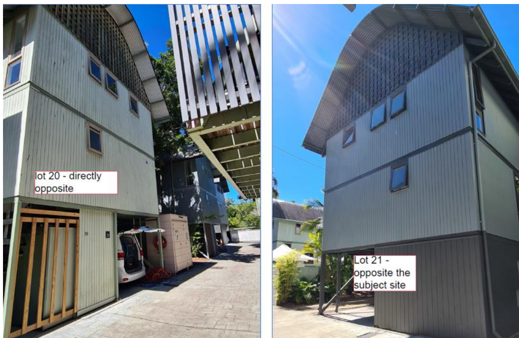
Figure 15 - Lots 20 and 21 have 4 small windows and are typical of other units on the eastern side of the internal driveway.
