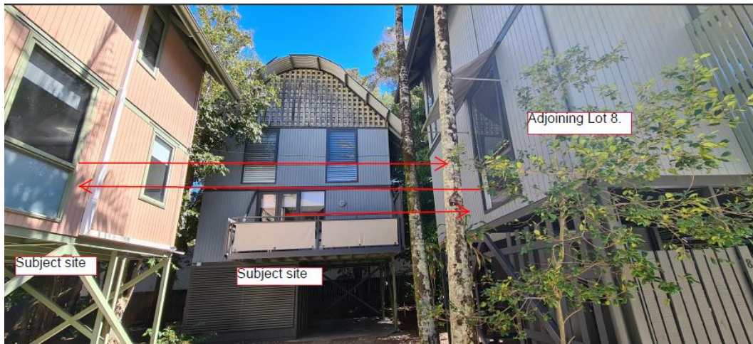
Figure 13 – Lot 8 privacy analysis, existing overlooking
