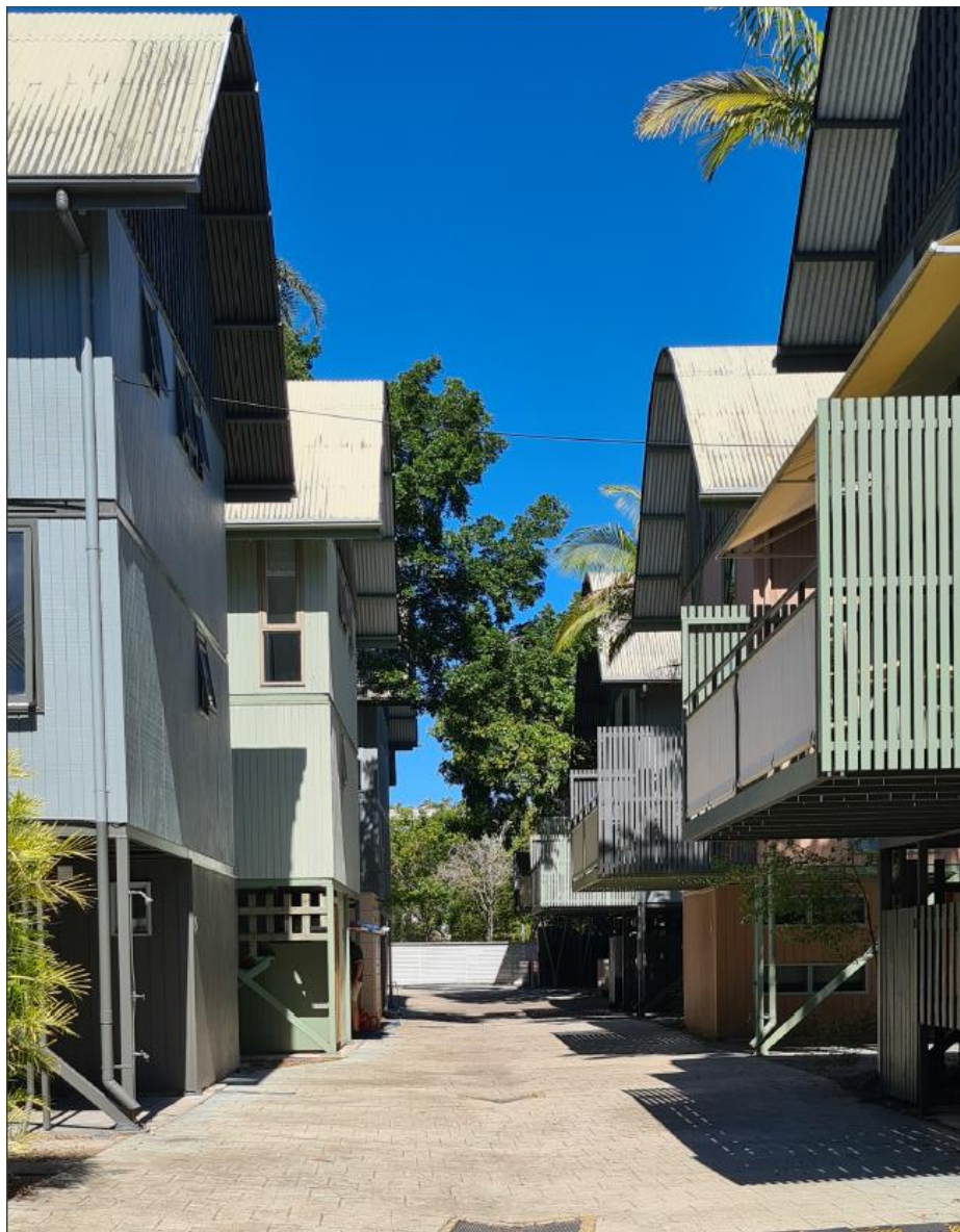
Figure 12 – Context of existing privacy and overlooking. Eastern side of the driveway on the left and the western side on the right of the image.
