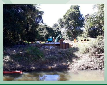
Precast concrete components are being used, with concrete deck units and kerbs ready to go and concrete headstocks and wingwalls being made next week. Steel fabrication of the bridge barrier is also under way.
