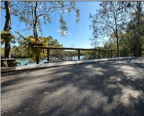
Reconstruction viewed from the road
