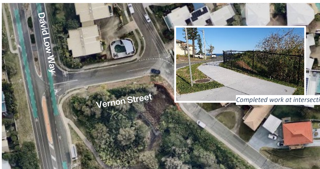
Location of damage at the intersection of Vernon and Sobraon streets
