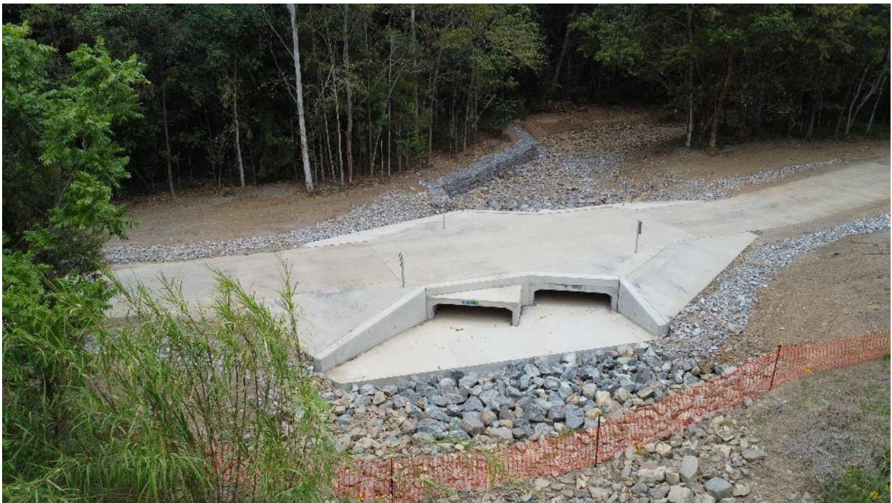
Completed reconstruction at site 2
