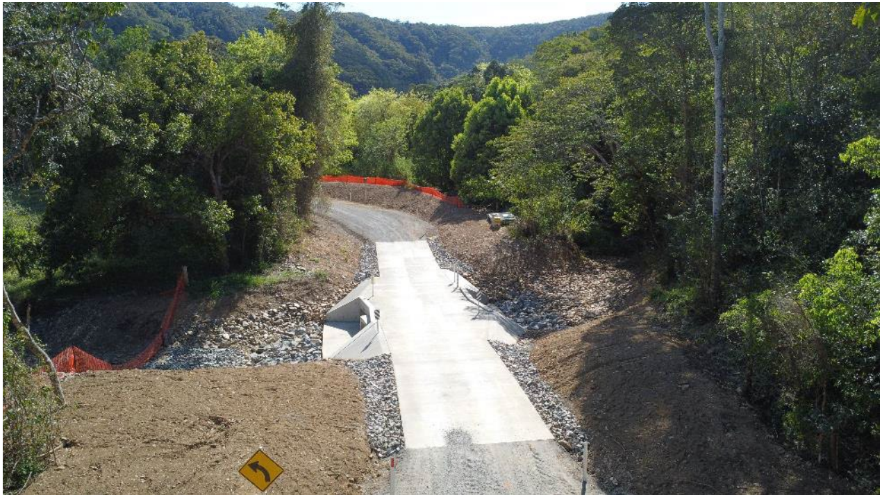
Completed reconstruction at site 1
