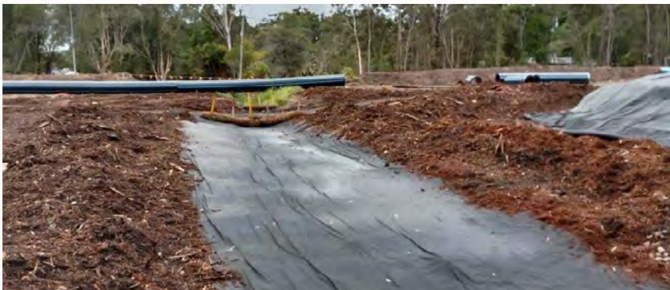
Tewantin bypass clean water diversion (image source Aiden Flannery).
