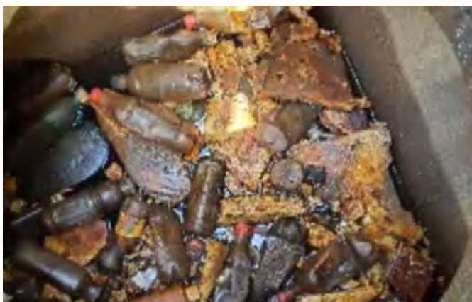
Rubbish accumulated in gross pollutant trap during audit (image source Sophie Blond)
