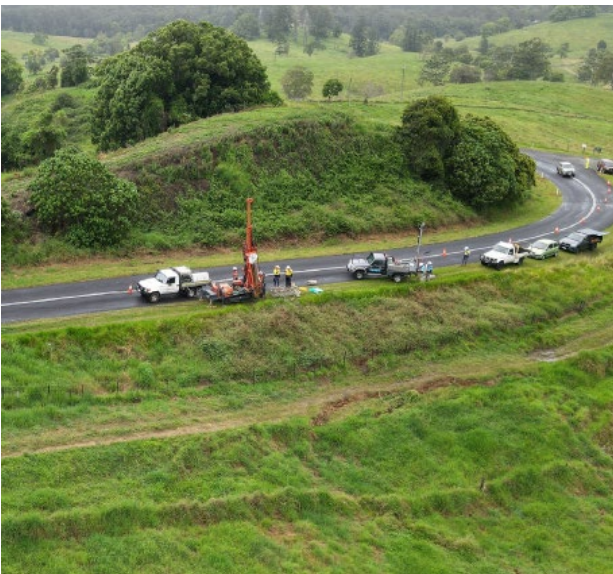
Geotechnical investigations on Cootharaba Road following landslide damage in February 2022.
