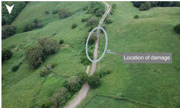
Aerial view showing location of damage on Simpsons Road
