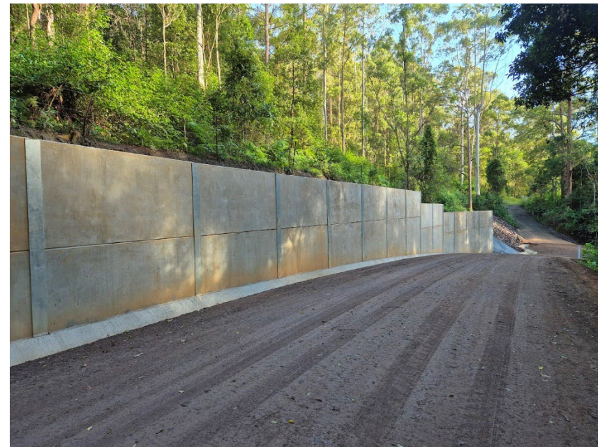
Completed reconstruction work and road re-opened to traffic.
