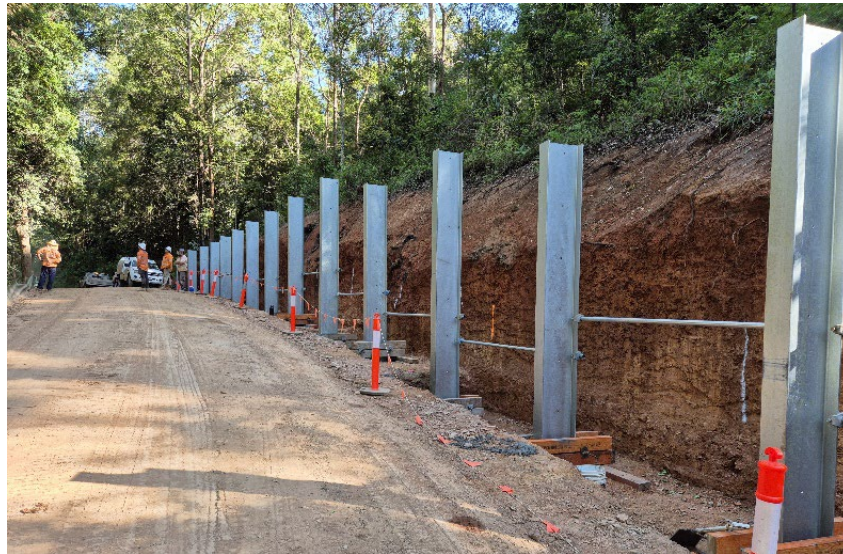
Supporting columns for retaining wall. These columns are 5.1m below ground.
