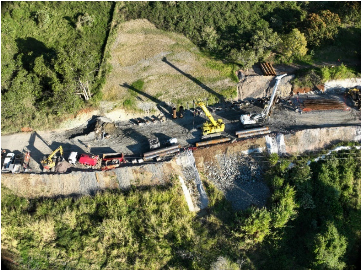
Drone footage of progress at Black Mountain Road – September 2024
