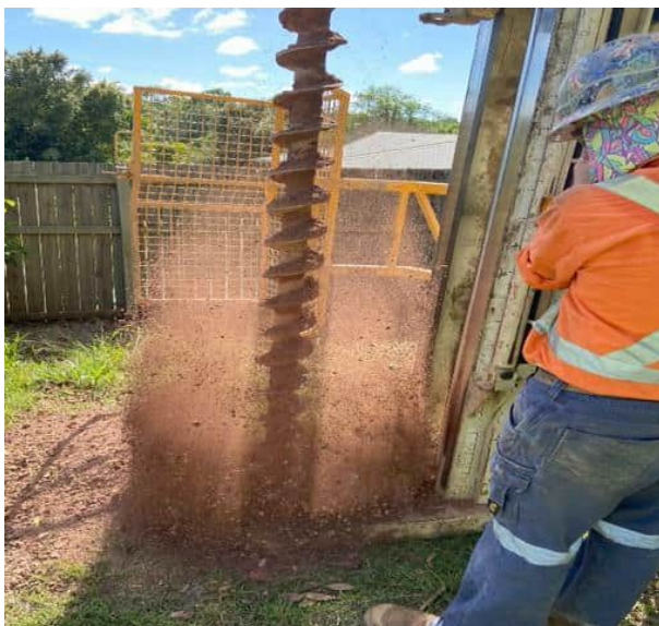
Photo 17 – drilling MB3 on 23/2/24
