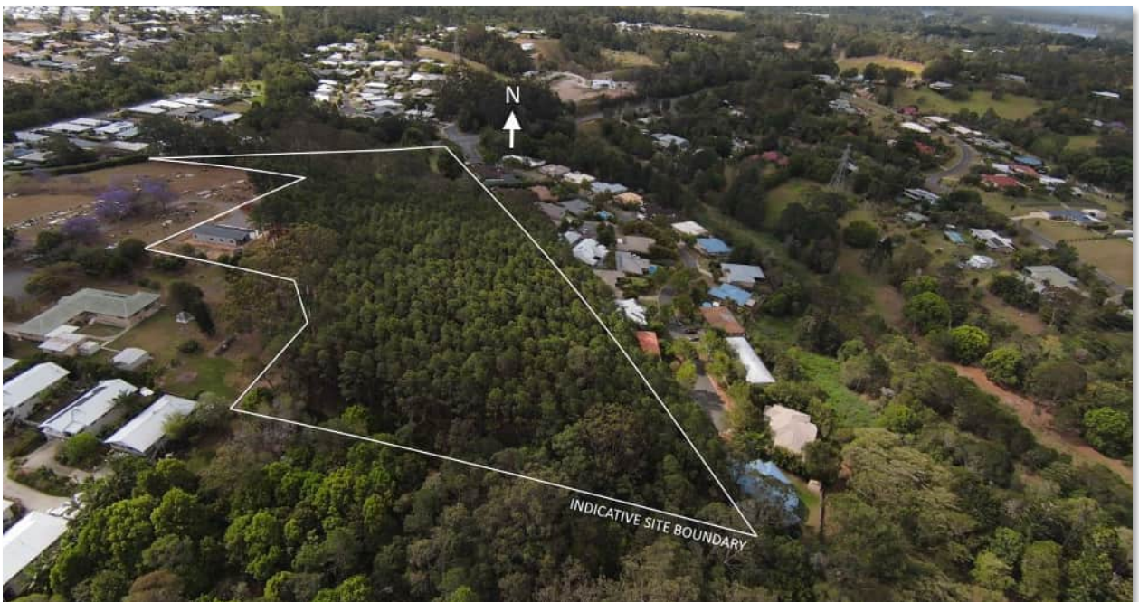
Photo 2 – Oblique view looking north 18/10/23
