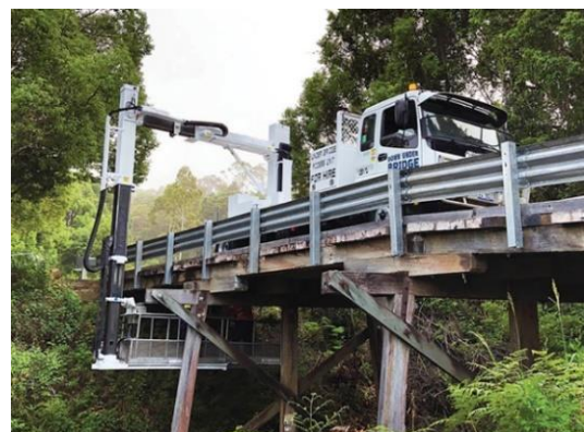
IMAGE: Typical Under Bridge Inspection Unit
